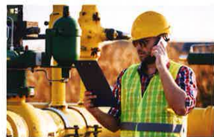
Mobile phones can act as an energy source and may ignite flammable vapours
