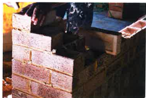
Clay bricks in use on a construction site
