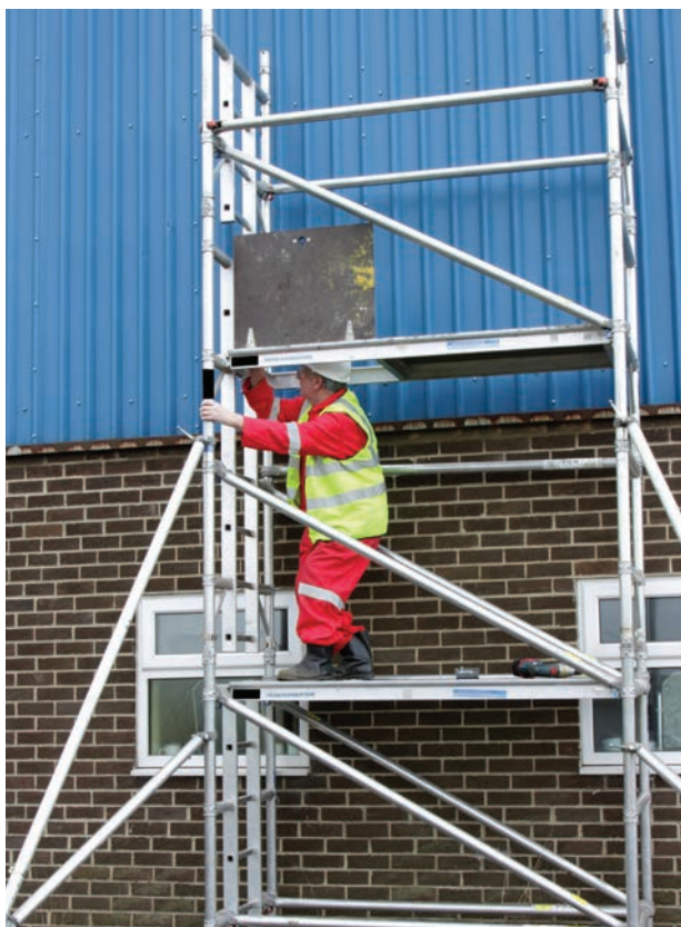
A worker gains entry to the top work platform of a tower scaffold.
