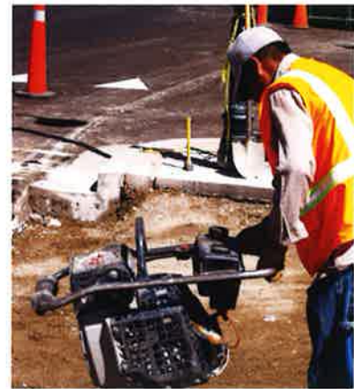
Compactors and other tools can generate a lot of vibration, which is then delivered into the hands and arms of the worker
