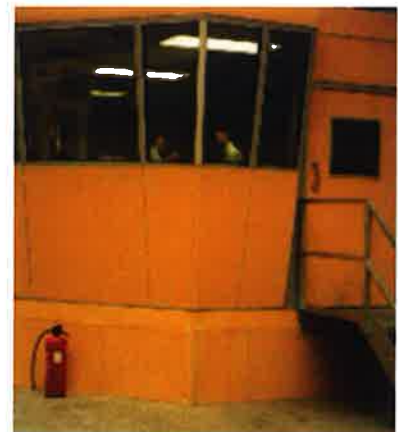
A noise refuge and control room Source: L108 Controlling noise at work (2nd ed.), HSE, 2005 ( www.hse.gov.uk/pubns/books/l108.htm )
