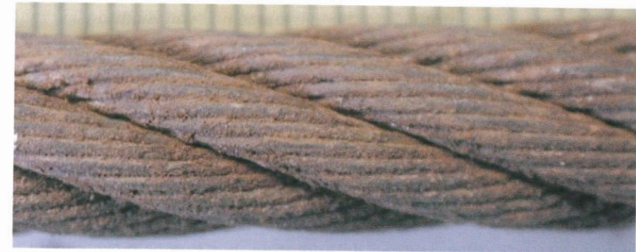
Wires rough to touch, general surface oxidation Rating: 20% towards discard
