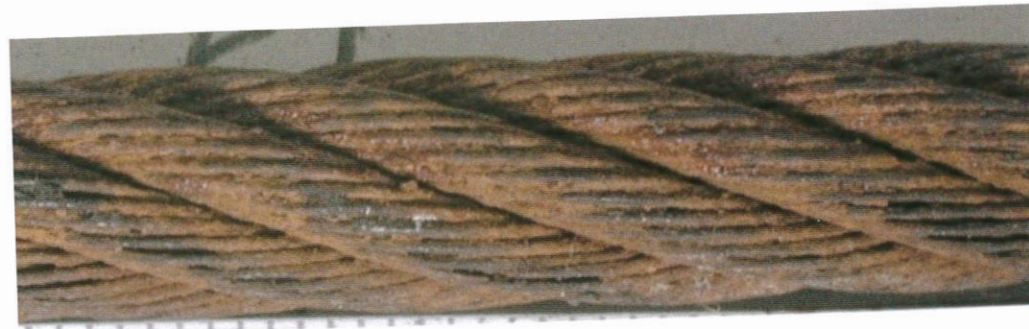
Surface heavily pitted and wires quite slack, gaps between wires Rating: Discard immediately
